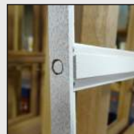
Muntins are doweled for added strength and support
