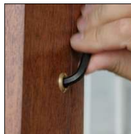
Screen/storm panel removal
