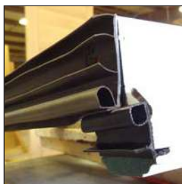
Astragal sweep on double door keeps water and air out
