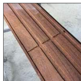
Weep systems under the double door sills to weep water away
