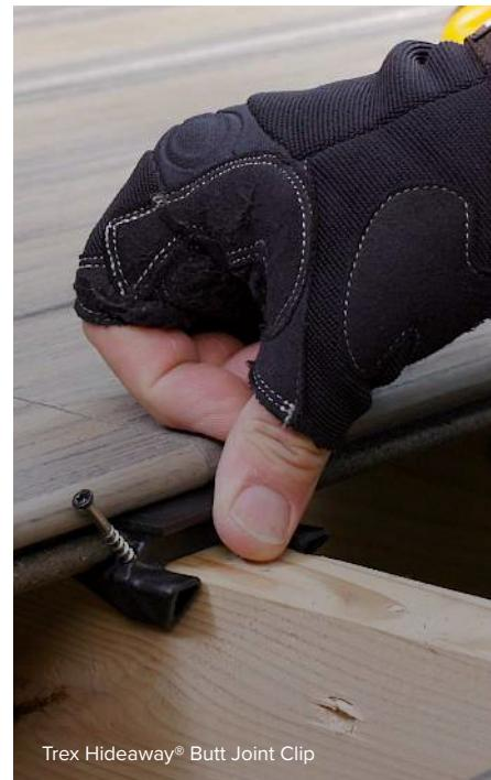
Trex Hideaway® Butt Joint Clip
